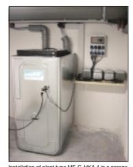
Installation of plant type MF-G-HKA 4 in a garage in combination with an existing septic tank
