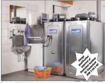
The plant type MF-HKA 4 for 4 inhabitants consists of two double-walled safety tanks and in a
