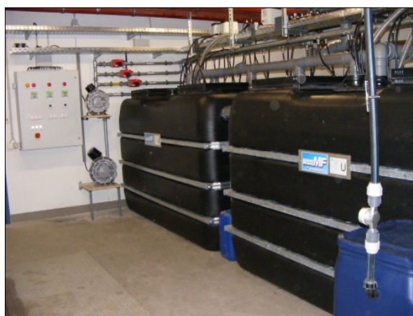
Small scale sewage treatment system
