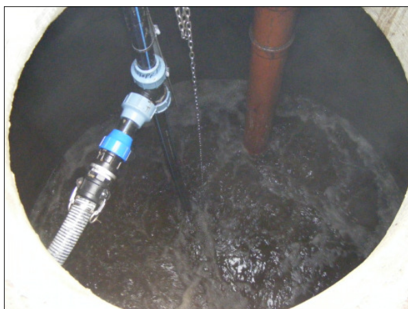
Septic tank with pumping unit
