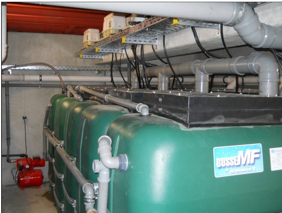
Waste water treatment system
