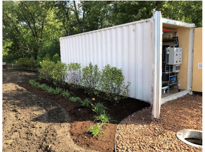
Exterior view of the container plant
