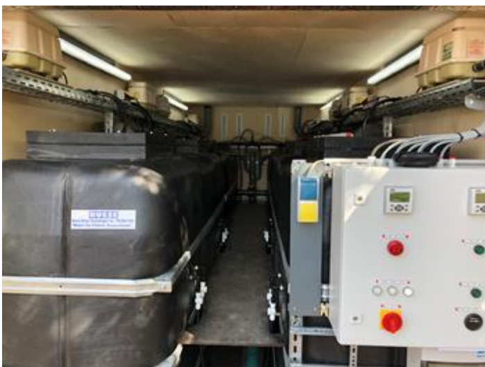
View into the interior of the container. A footbridge between the rows of tanks enables trouble-free work at the blowers fixed above the tanks. It also guarantees access to the membrane modules, which are installed in the tanks.
